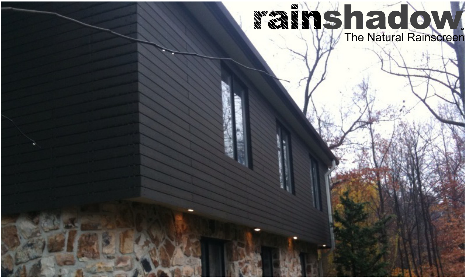
Private Residence, Philadelphia, PA , Arch: Point B Fabrication
