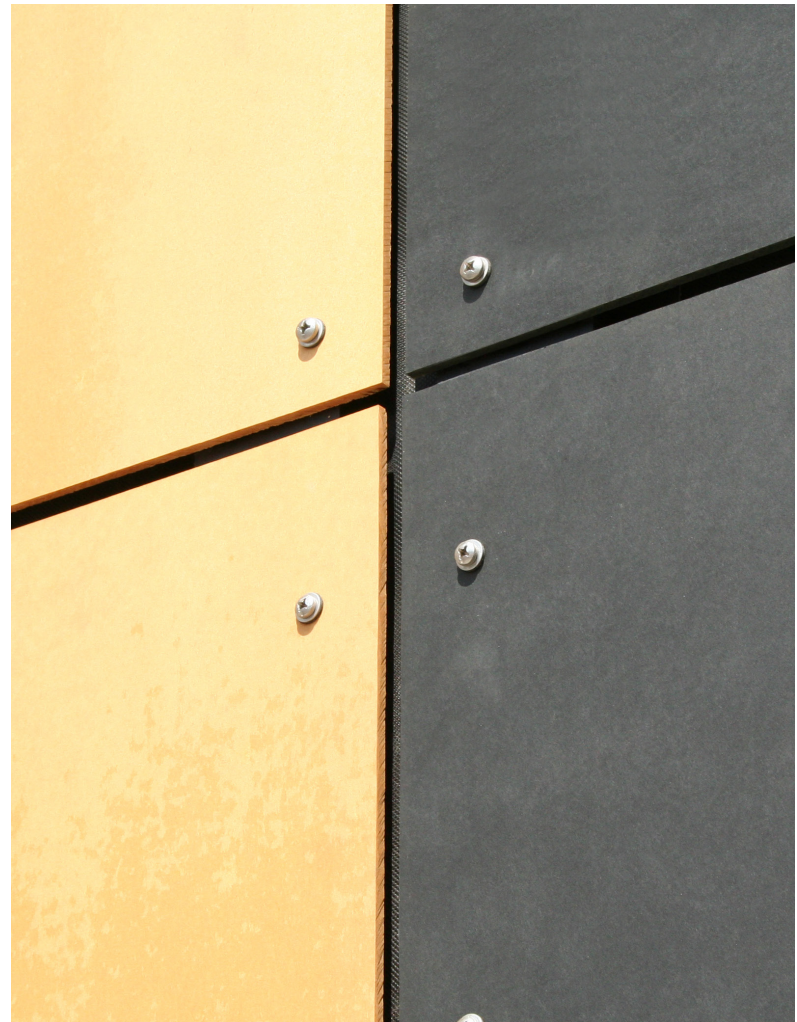
Alley 24, Seattle, WA , Arch: NBBJ
